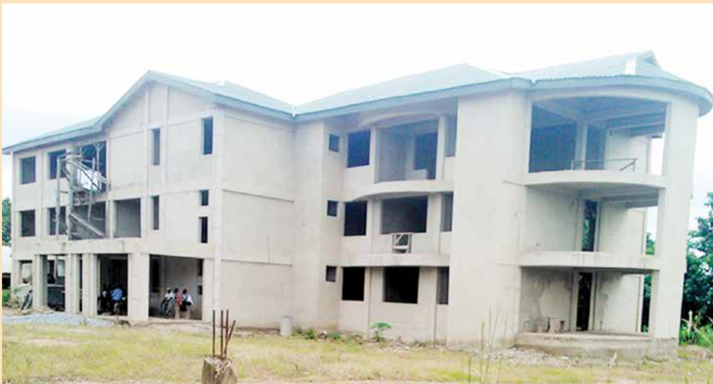
3-Storey Office Accommodation (Ongoing)
