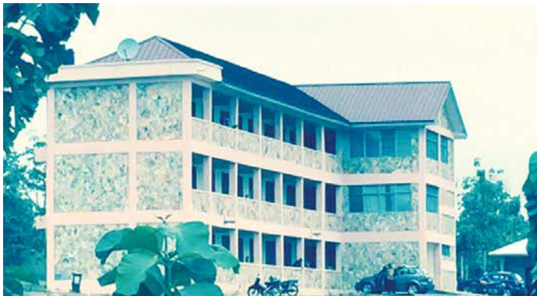
Kintampo South District Assembly Office Block
