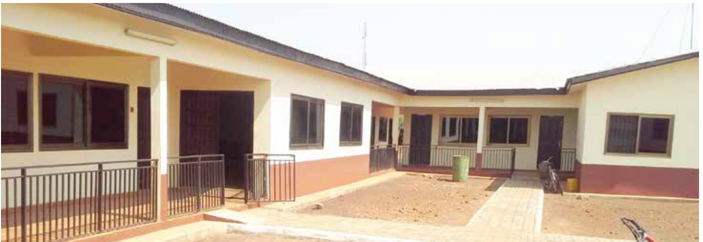
Newly Constructed Assembly Office Complex at Bunkpurugu
