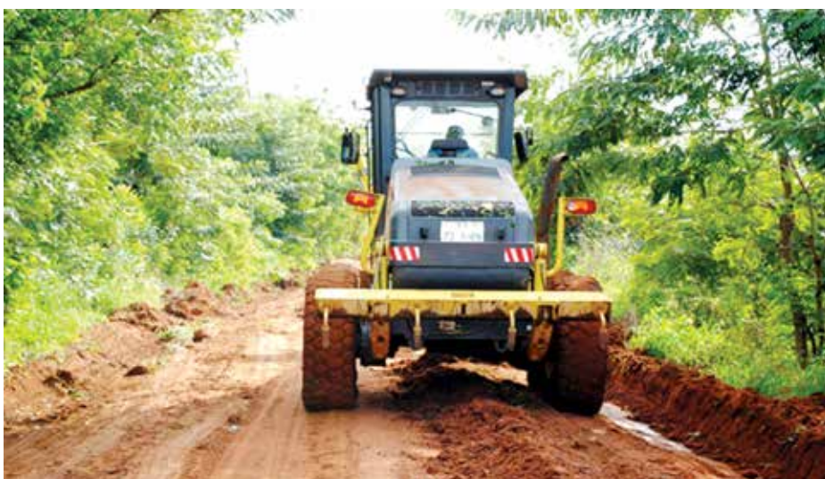
Regravelling of the Asesewa to Brepaw Feeder Road
