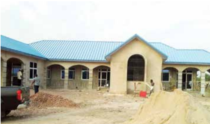
Construction of DCE bungalow at Tolon
