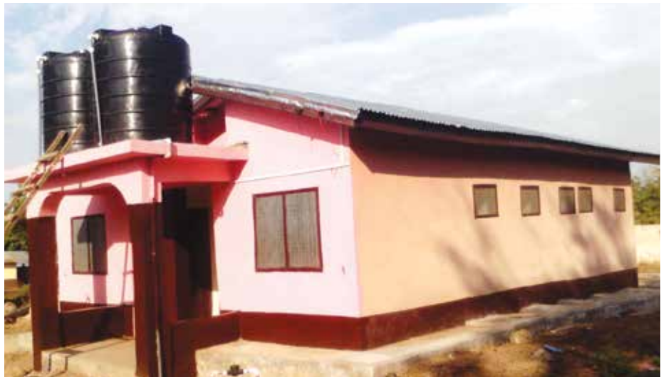
construction of 5-seater toilet with over head tanks at Donkorkrom
